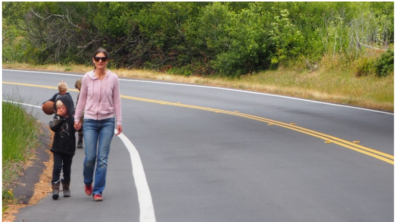
Figure 10: A minimum shoulder on Highway 1 near Elk, CA
