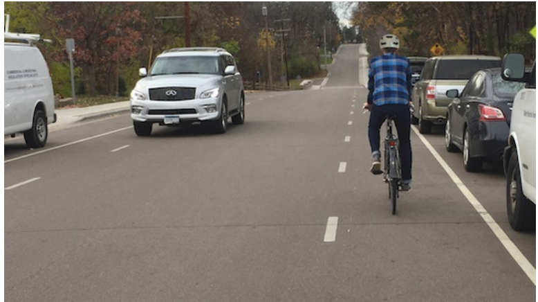
Figure 11: An advisory shoulder in Edina, MN showing vehicle shifting to give additional room for cyclist; Source: Small Town and Rural Design Guide
