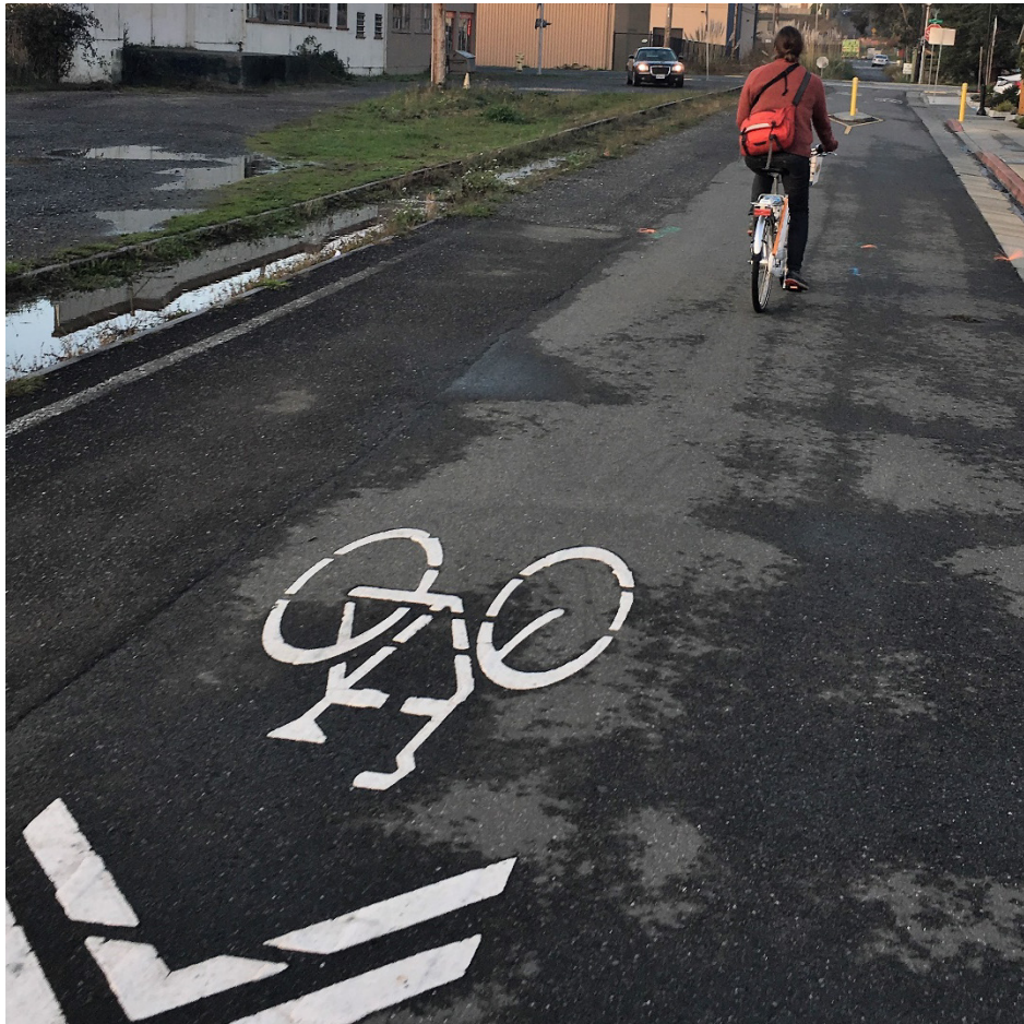
Figure 8: A Class III Bikeway with sharrow on L Street
