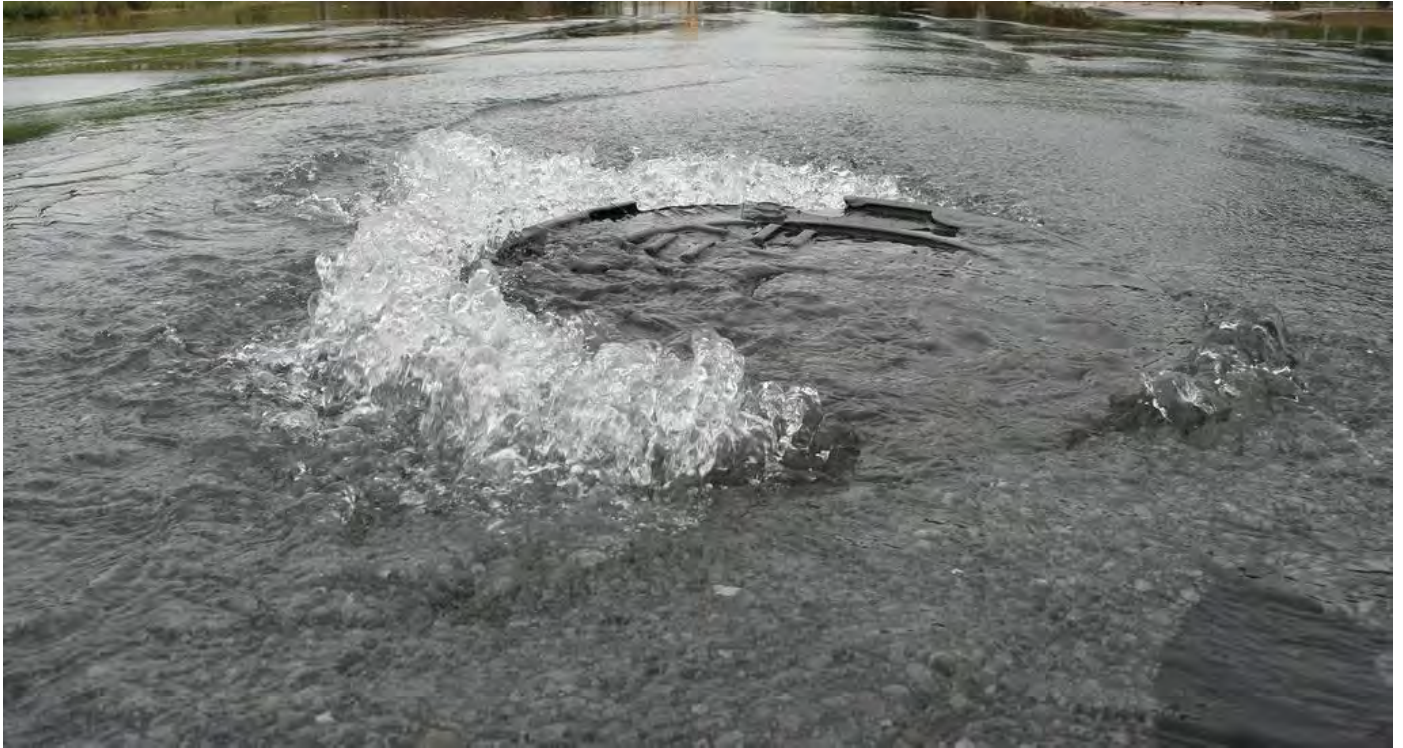
Figure 7 Example of Inundated Manhole Flooding Collection System
