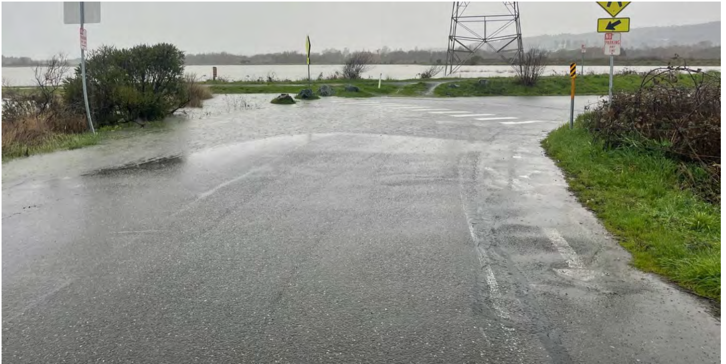
Figure 24 10.03-foot NAVD88 Water Level overtopping South I St into Hauser Marsh on January 3 rd , 2026.
