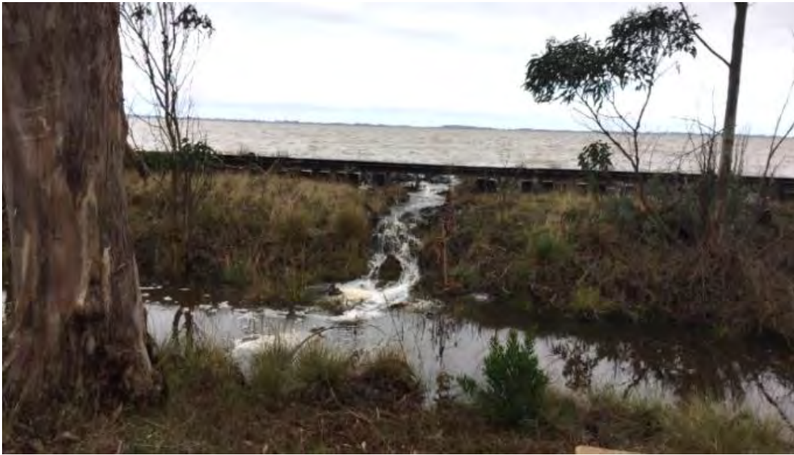
Figure 19 Observed erosion due to overtopping of fill prism.
