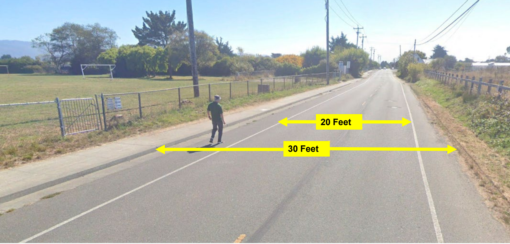
Janes Road facing south. The sidewalk terminates at the St. Mary Church south parking lot. Janes Road has sufficient traffic volume and speed to warrant a continuous walkway that extends northward to Foster Avenue and facilities to accommodate bicyclists.
