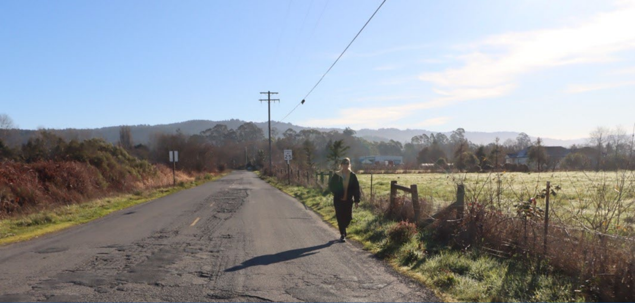
Foster Avenue, between Janes Road and Q Street, is approximately 20-22 feet wide with no shoulders and poor pavement conditions. While traffic volumes are generally light, they increase significantly during school pick-up and drop-off times. Additionally, the road serves as a truck route to farmland to the west.
