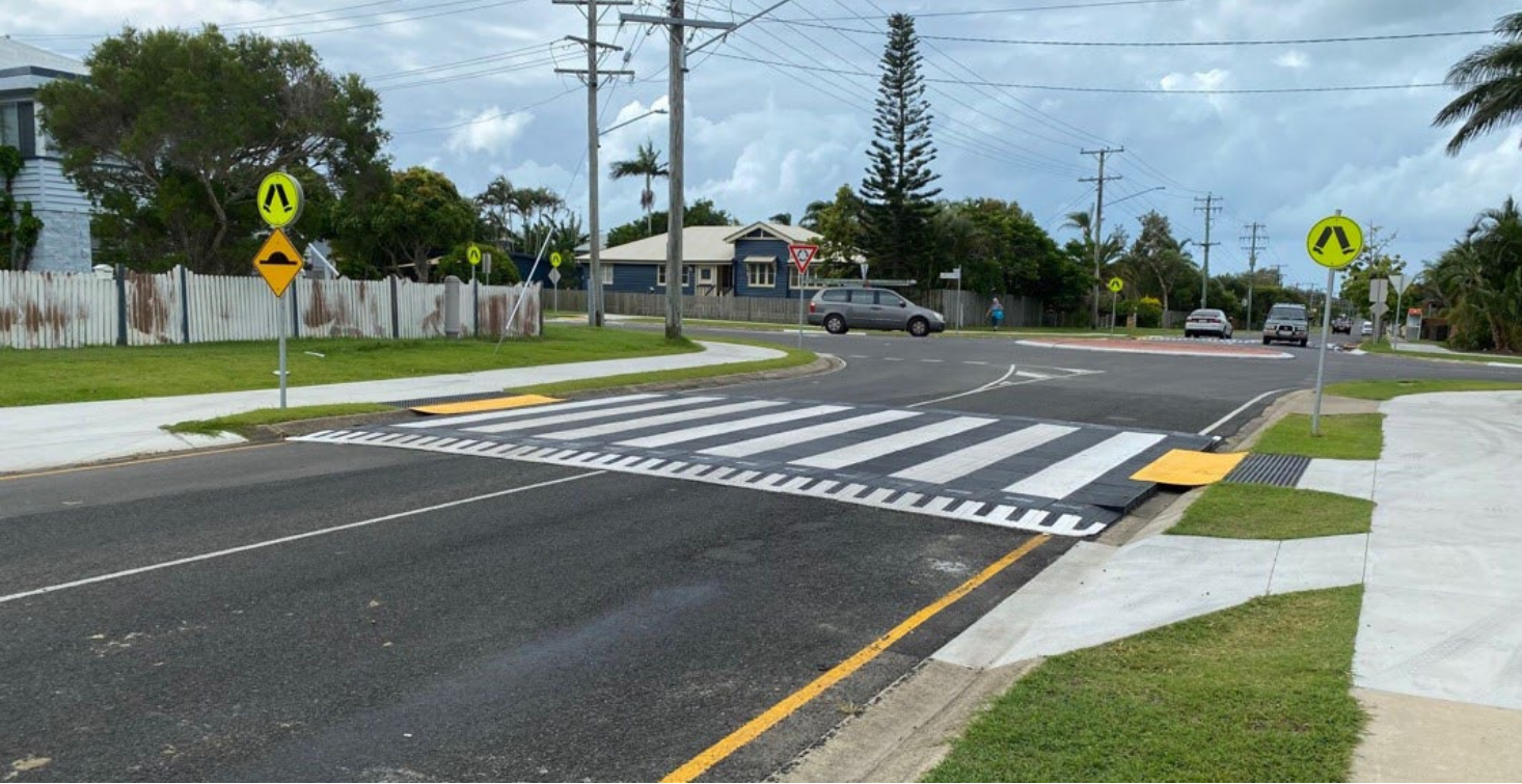
Quick-build raised crosswalk and roundabout with modular rubber components in Urgan, Australia.
