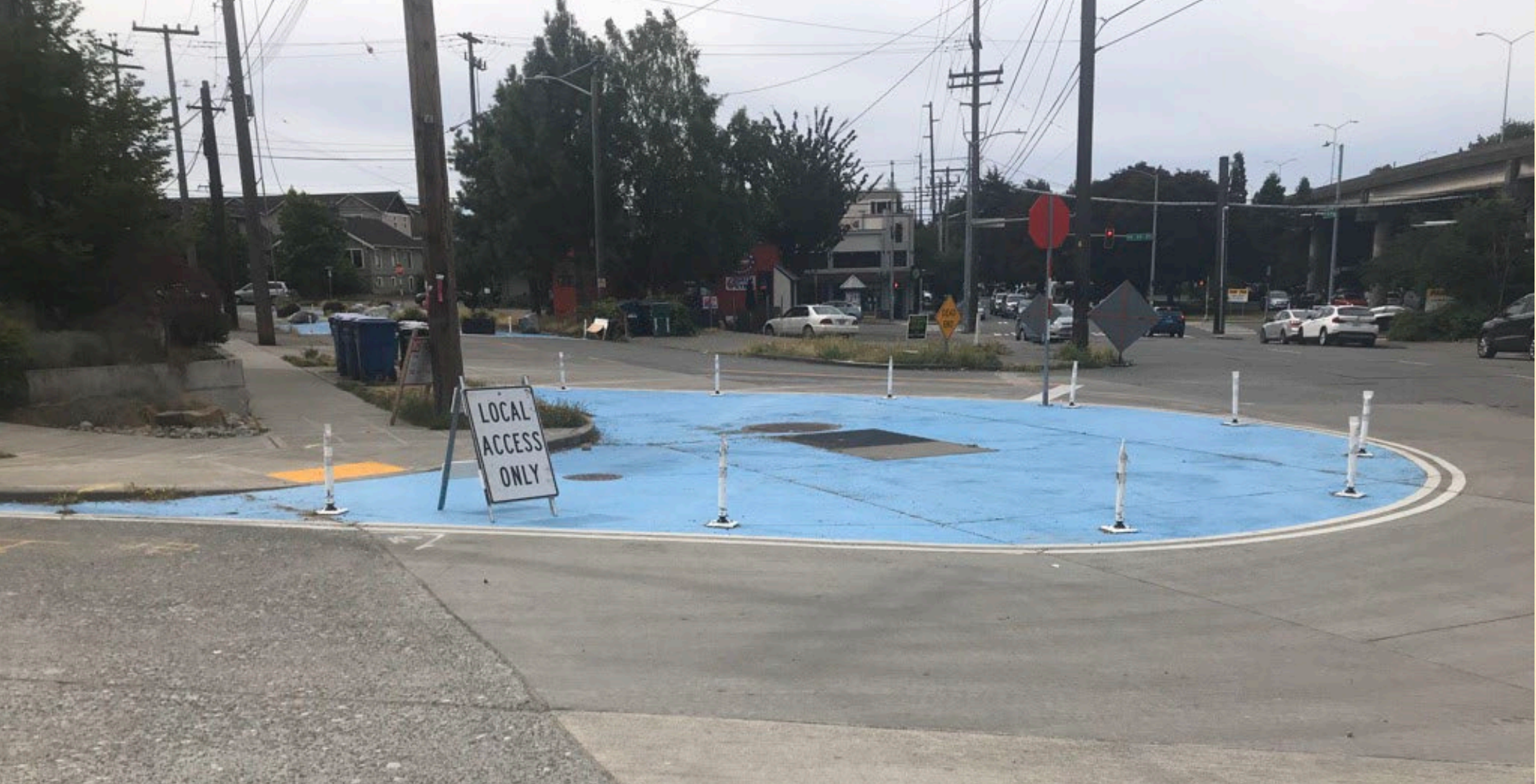
Quick-Build projects (paint and soft posts or street furniture) can be completed for under $5,000. These solutions can be placed and evaluated either short term, or for multiple years, until permanent funds are budgeted.
