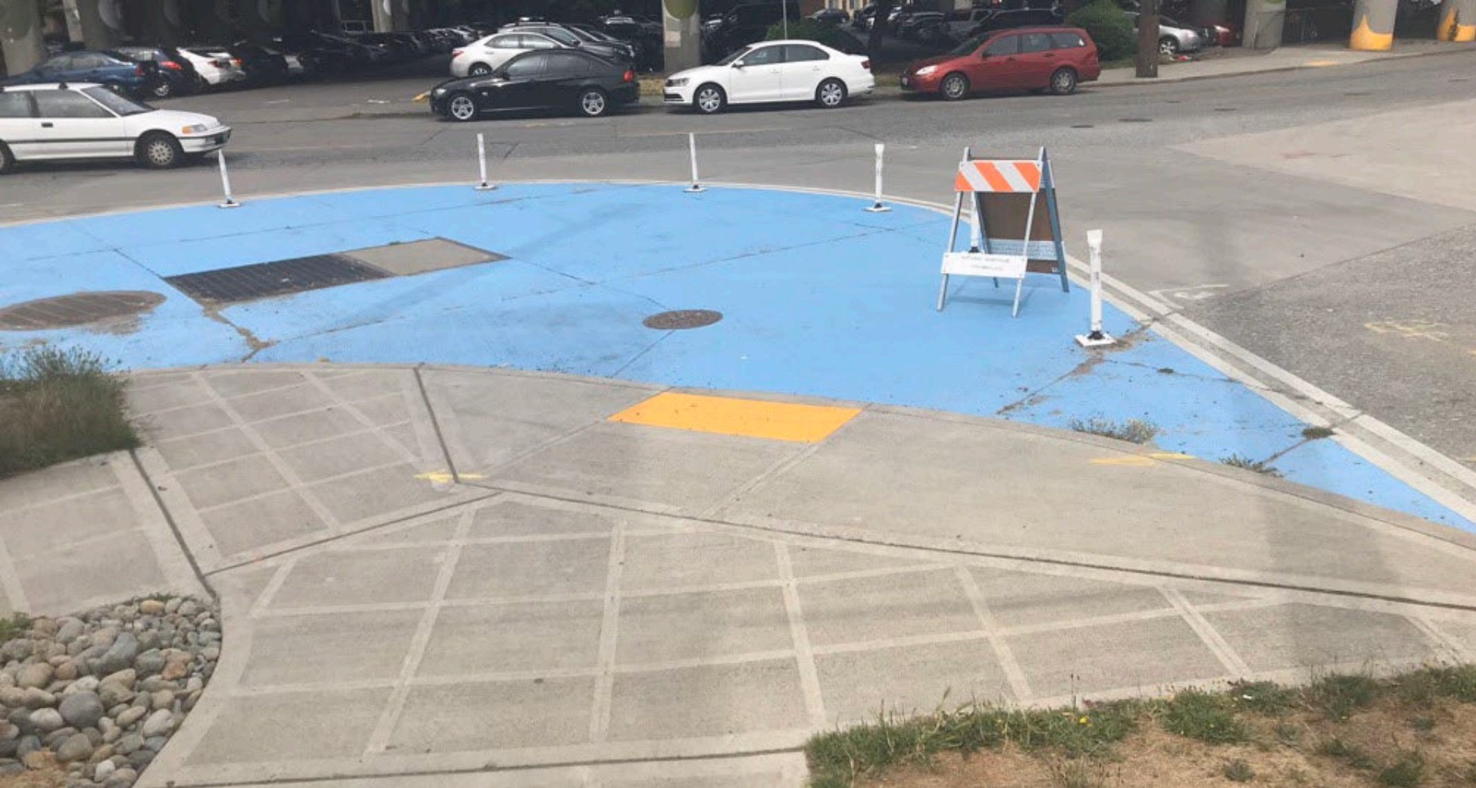
Quick-Build projects (paint and soft posts or street furniture) can be completed for under $5,000. These solutions can be placed
