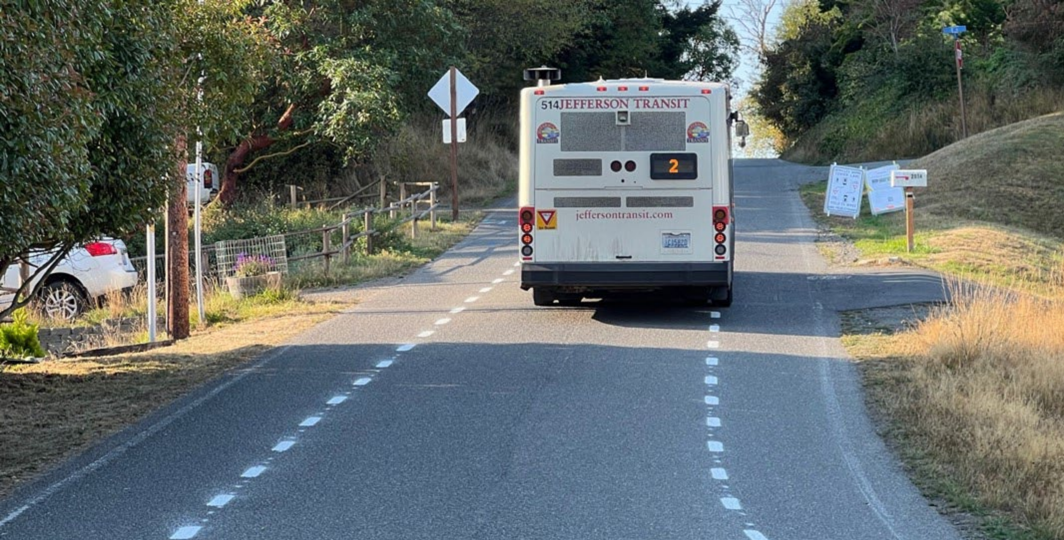
An example Edge Lane Road (Port Townsend, WA) Two-way Edge Lane Roads typically bring down speeds 2-7 mph, and increase safety for driving, walking and bicycling. Note with ELRs sight lines are improved for intersections and driveways.
