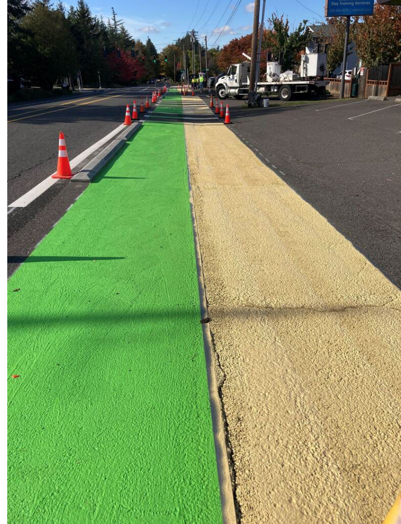
Striped walk & bikeway with curb protection under construction in Portland, Oregon
