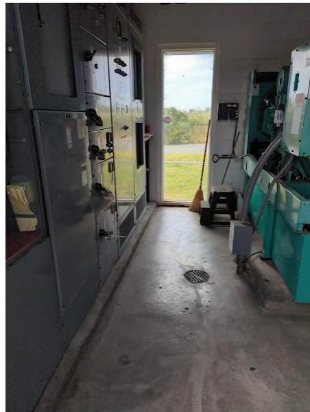
Figure 21 Typical lift station components consisting of A) lift station building on concrete slab B) lift station cabinet on concrete slab C) electrical panels and D) electrical panels and backup generators.
