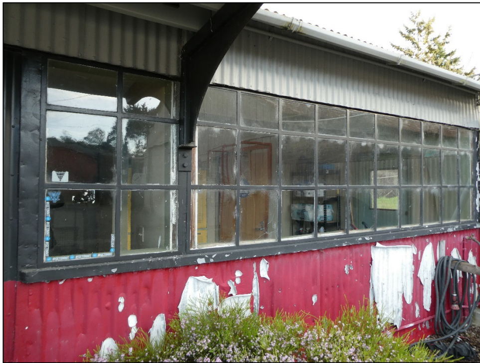
Photograph 6. Fixed steel-frame windows on Building A, camera facing north, March 21, 2024.
