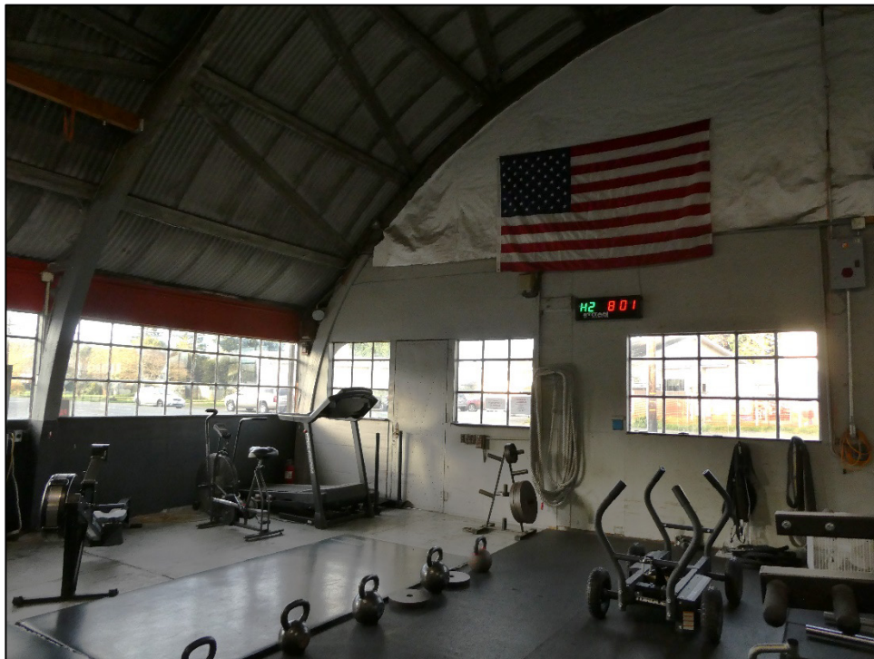
Photograph 4. Interior view of Building A showing laminated-wood trusses. Camera facing south, March 21, 2024.
