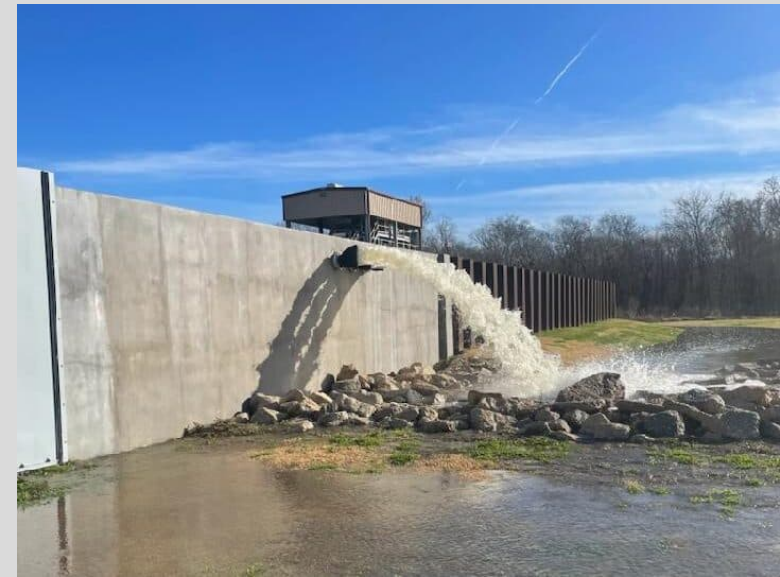
Concrete wall and sheetpile protection at Liberty, Texas – FEMA funded coastal hurricane storm surge flood mitigation.
