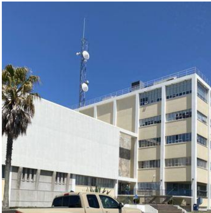
Telecommunications equipment on top of the Humboldt County courthouse building — a tower on top of a 5-story building.
