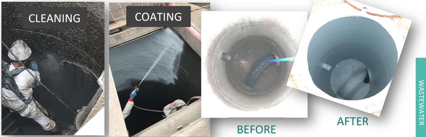
Annual Manhole and sewer line rehabilitation/replacement project. Typical projects may include cleaning and coating the inside of manholes or lift stations (to reduce I&I), and/or reconstruction of portions of our sewer system to repair damaged sections or correct problems which require regular maintenance.
