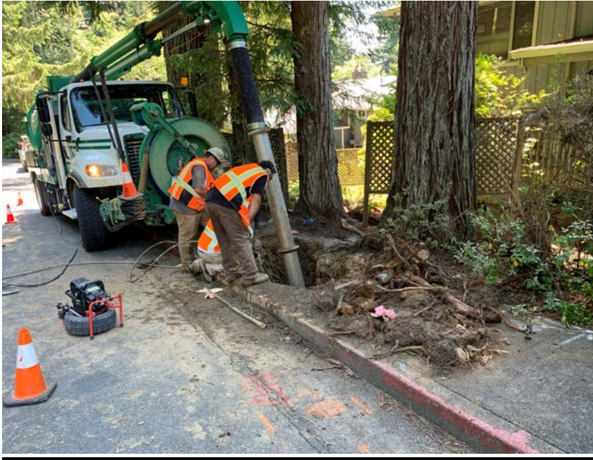
Utilities Crew working to remove roots affecting distribution lines
