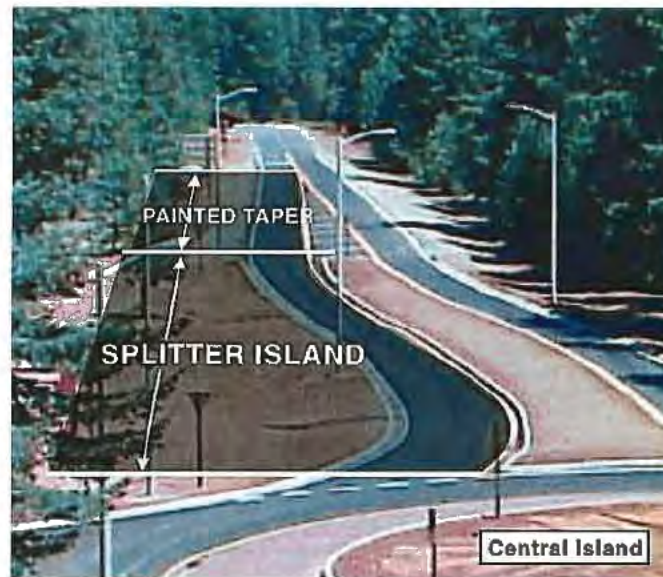
Figure 29. Annotated Photograph of Roundabout in Kittitas County, Washington, Showing Painted Taper and Splitter Island Incorporating Geometric Reverse Curves to Transition Driver Speeds.
