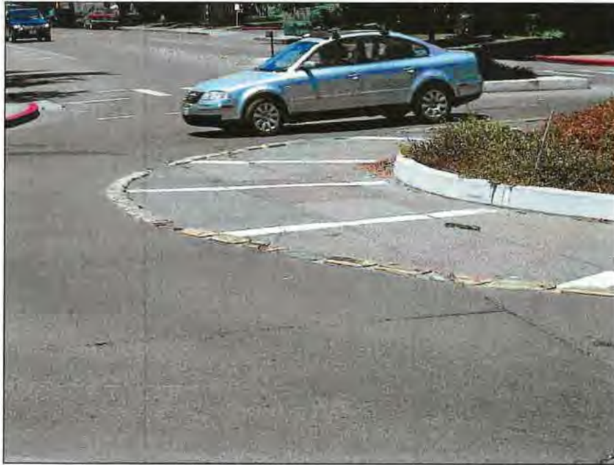
Figure 3. Inadequate Apron Design and Use at Anderson Road/Alvarado Avenue Roundabout in Davis
