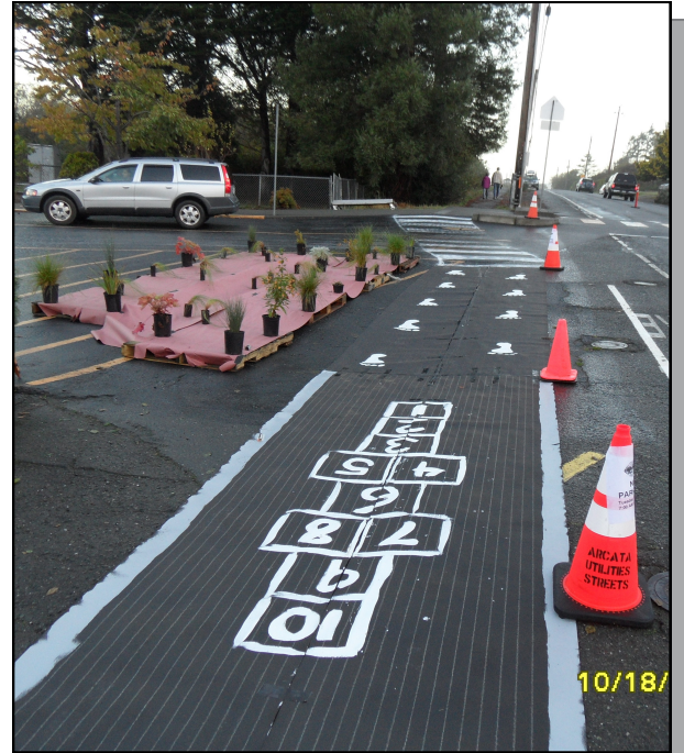
Pop-up infrastructure installation in front of the Jacoby Creek School, demonstrating a separated path, new crosswalk, parking alterations, and landscaped "bulb-ins."
