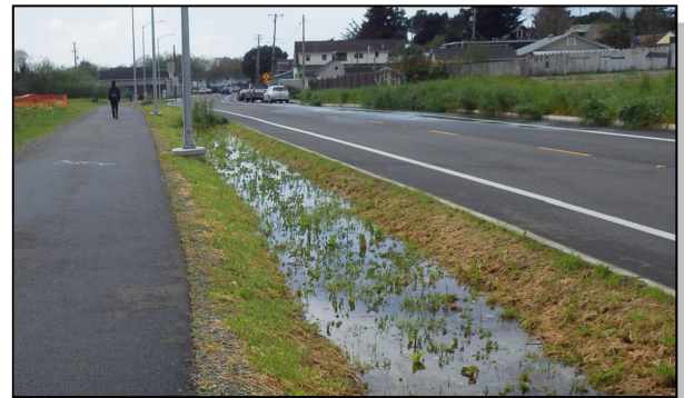
Vegetated swale at the City's recent Foster Avenue extension project.
