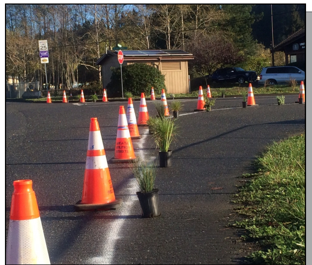
Pop-up infrastructure installation at intersection of Jacoby Creek Road and Old Arcata Road, demonstrating a narrowed intersection with planted areas.
