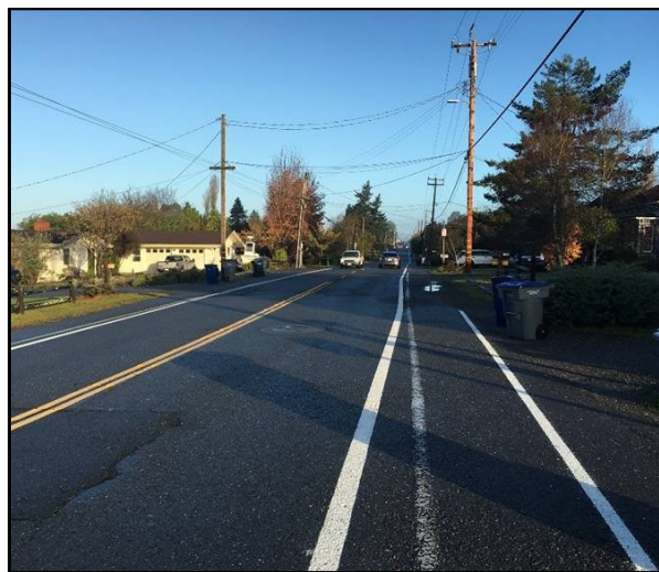
Recent upgrades performed by the City include roadway patching and restriping.
