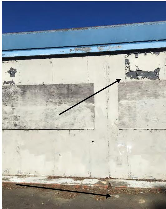
Photo 7: View of peeling paint and stained concrete at former Ericson Garage, adjoining northern extent of Project alignment; facing north.
