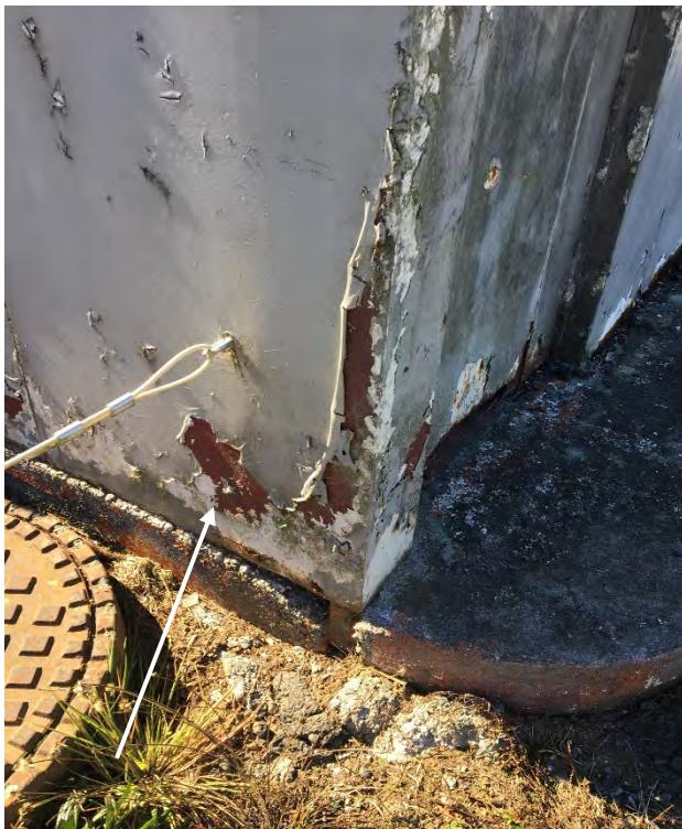
Photo 5: View of peeling paint on former Ericson Garage adjoining northern extent of Project alignment; facing south.
