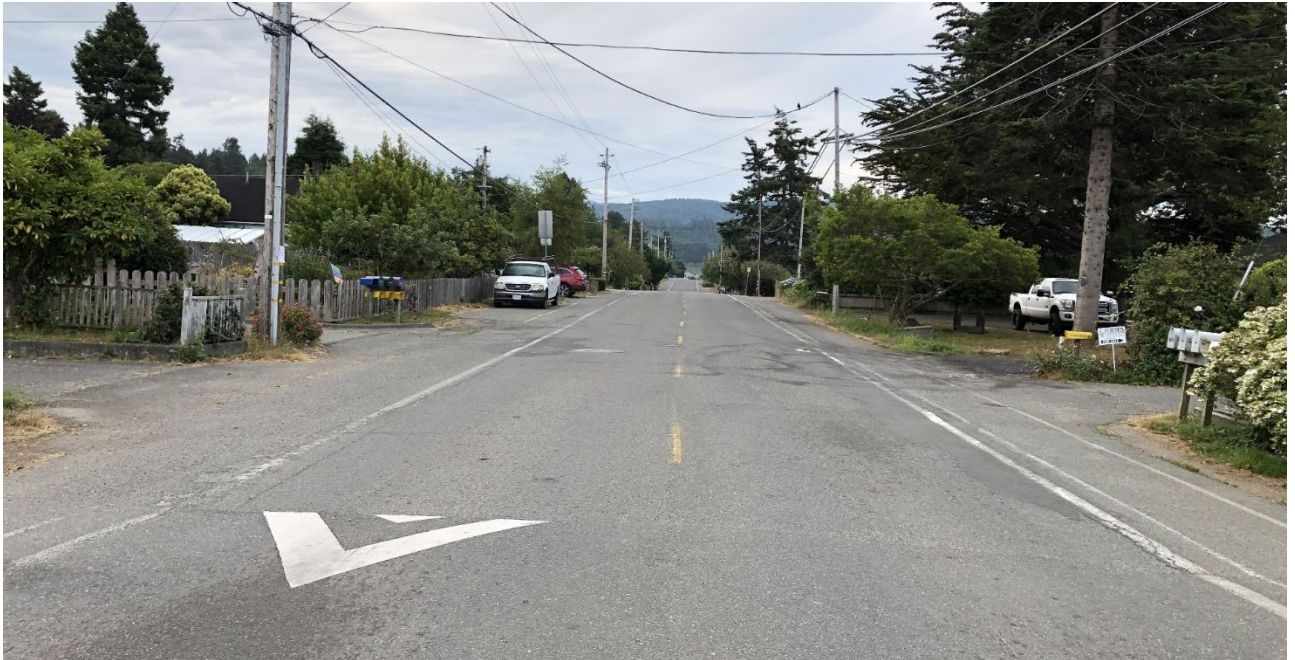
Exhibit 1: General Existing Conditions of the Old Arcata Road Streetscape Showing Deteriorated Paving, Striping, and Bicycle Lanes.
