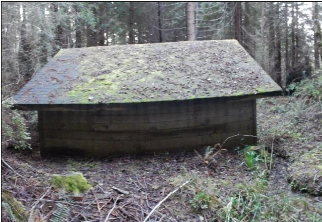
Figure 3. Active domestic surface water intake and diversion infrastructure identified as “Large wooden water building” on Map 2.
