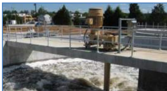
Excell® Aerator at 30Hz (20% power; 80% turndown)
