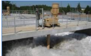
Excell® Aerator at 60Hz (100% power; 0% turndown)
