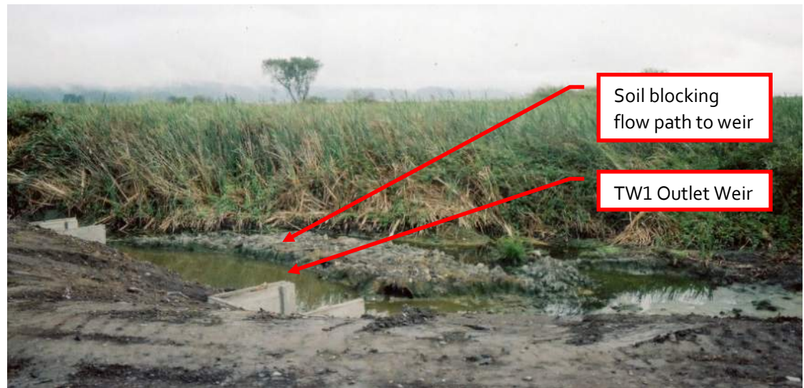
Figure 4.8 Soil Obstructing Flow at TW 1 Outlet Weirs (Photo courtesy of Gearheart, 2018)
