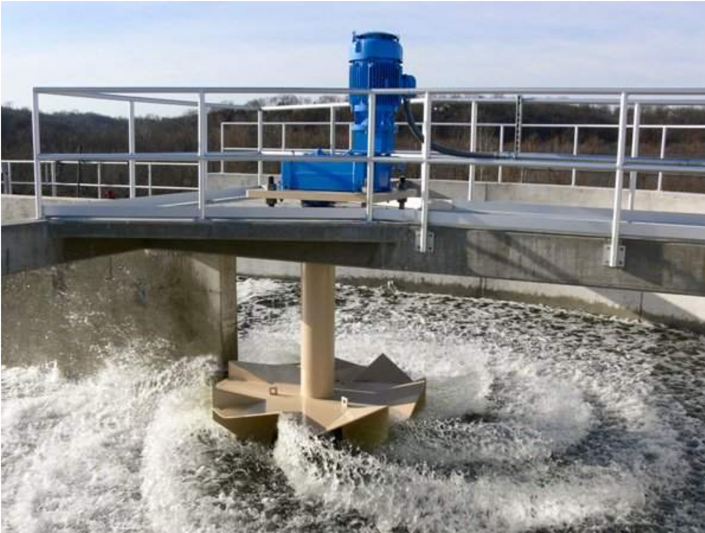
Figure 5.6 Surface Aerator
