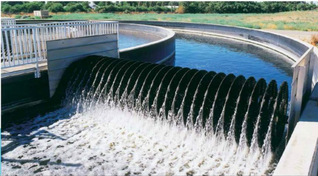
Figure 5.5 Proprietary Disk Aerator
