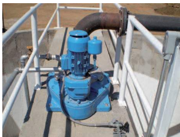
Reliable bull gear drive for the stirrer
