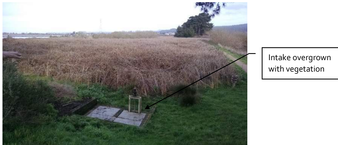
Figure 4.15 EWPS Intake Overgrown with Vegetation
